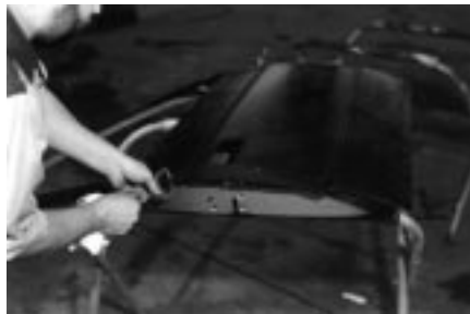
Figure 4—Attach clamps to the mating flanges to hold the panel in place while the adhesive is curing. (Courtesy of Kent Industries)
